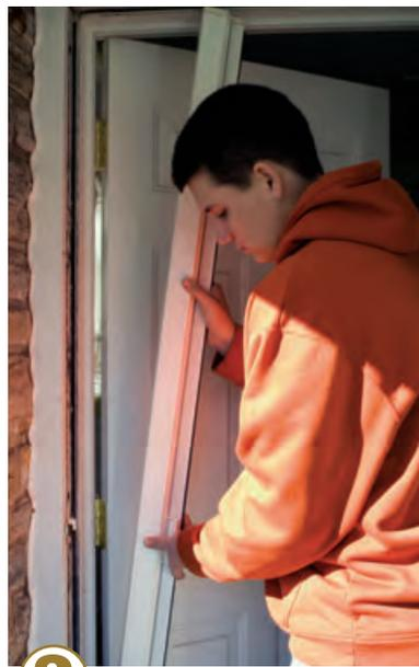
**2** Snap the storage cassette into the mounting clips, then mark its position on the side jambs with a sharp pencil.
