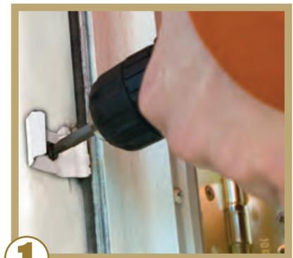
**1** Fasten two metal mounting clips to the side jamb head casing over the doorway. Use one screw per clip.
