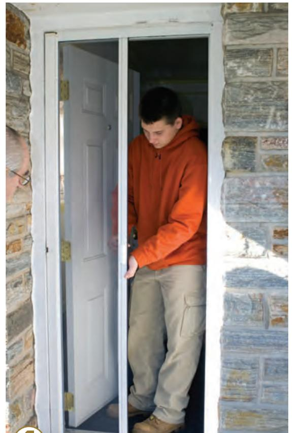
**4** Test the screen door by pulling on the handle. It should glide without hesitation.
